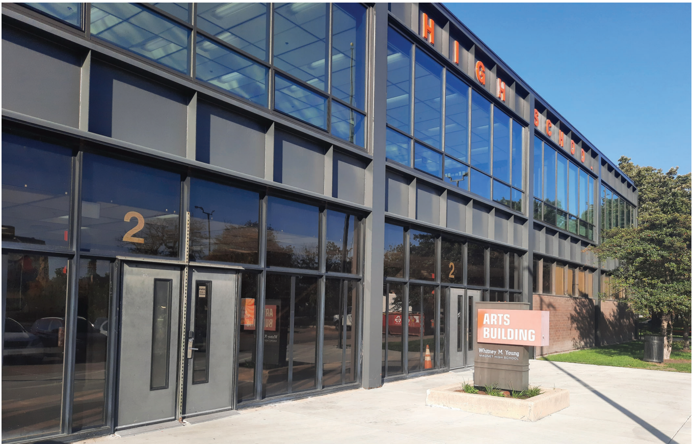
Top: Building A NE View Bottom: Bldg C Upper Floor View from SW
