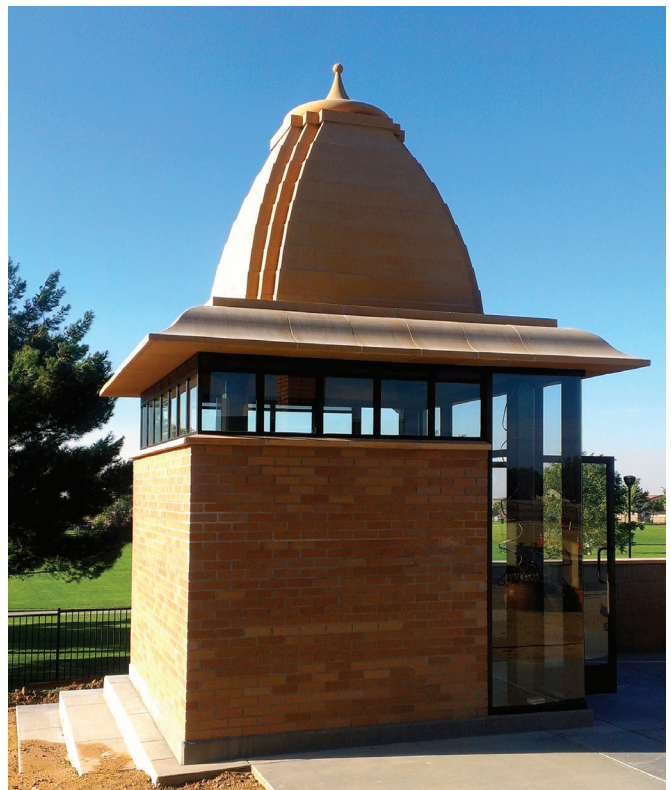
Top: View of main hall from south east Bottom L&R: View of temple NW and Navagraha
