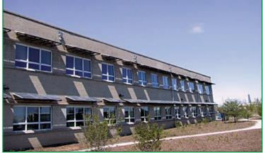
**figure 5.** BIPV in window awnings for Chicago Center for Green Technology.
