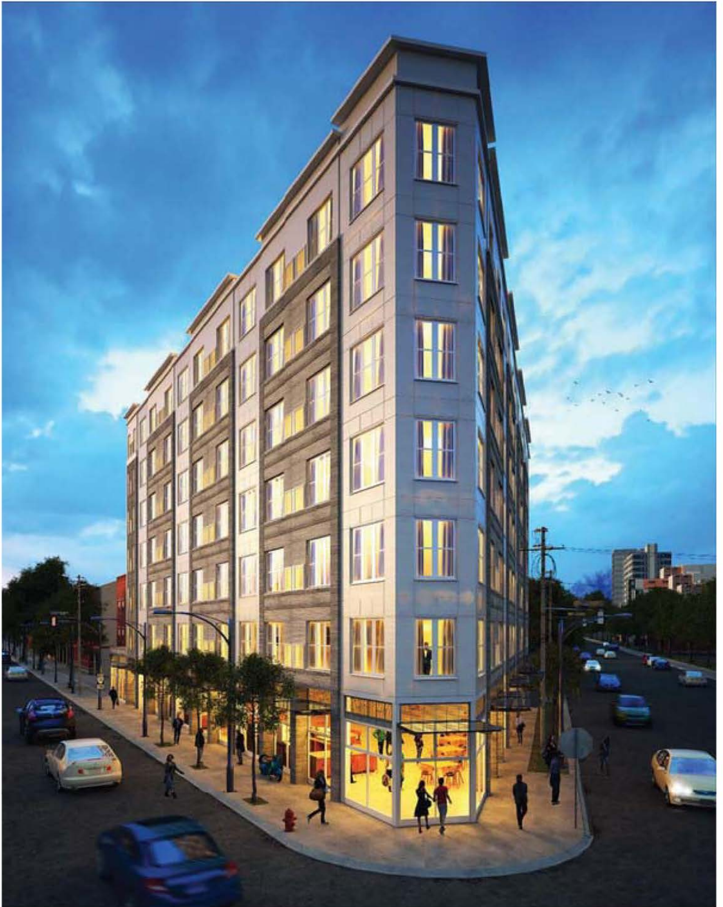
The seven-story project will be clad in a combination of brick and fiber cement. | CSA Partners Ltd.
